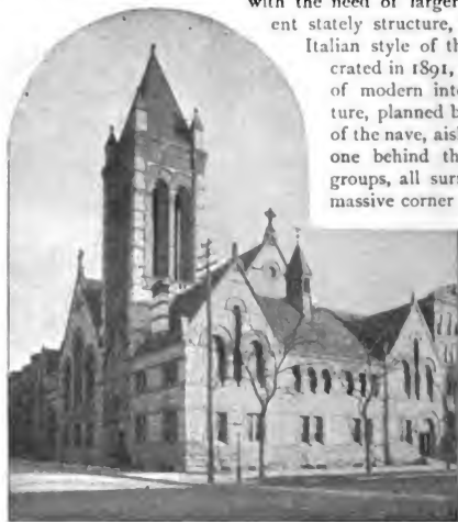
CHURCH OF THE HOLY TRINITY, PROTESTANT EPISCOPAL, LENOX AVENUE AND WEST 1220 STREET.
